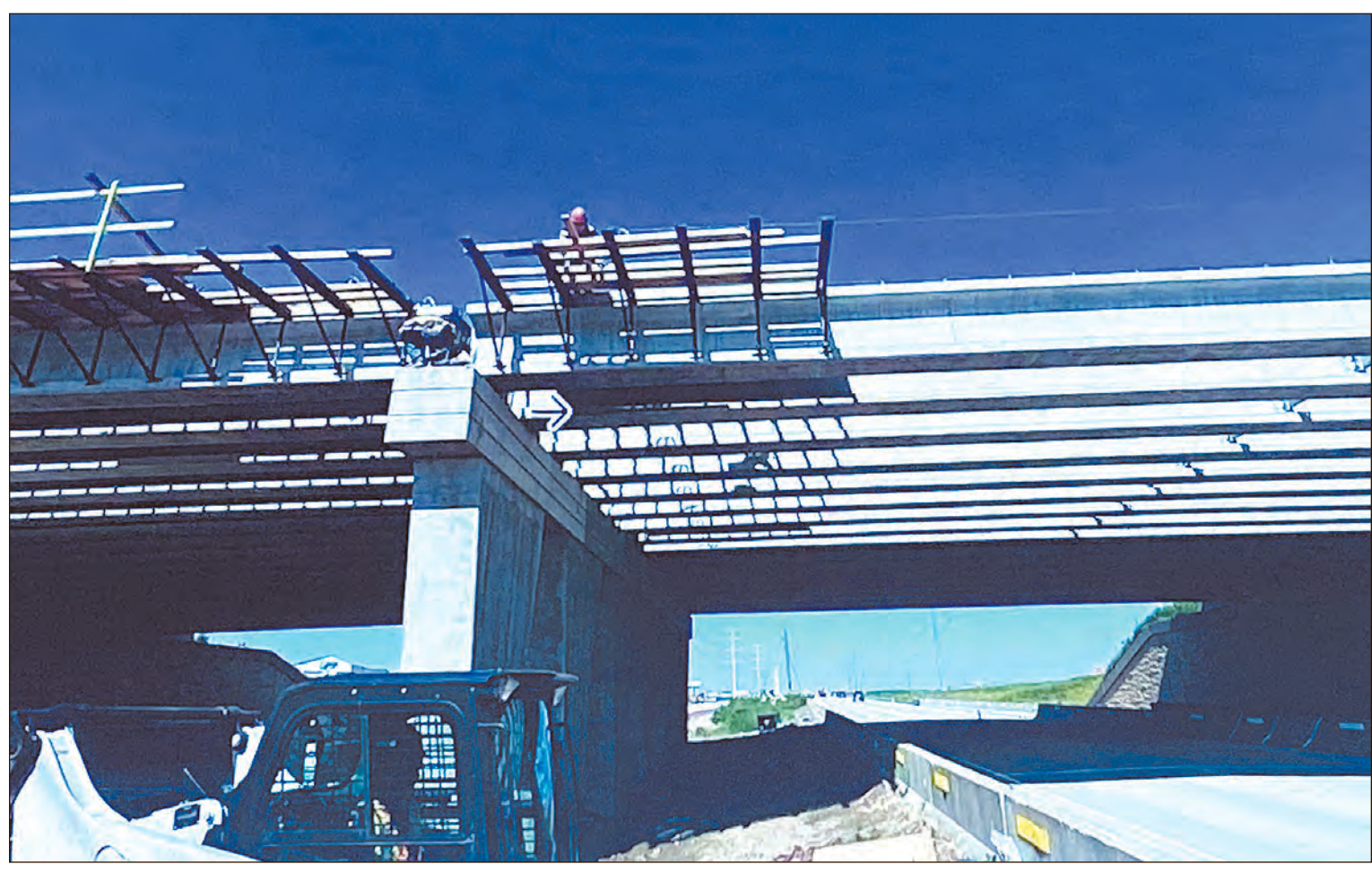
T&R Contracting, Inc. of Sioux Falls, continues to work toward near completion of Exit 406 at Brandon. This photo shows exit bridge form work in July.
