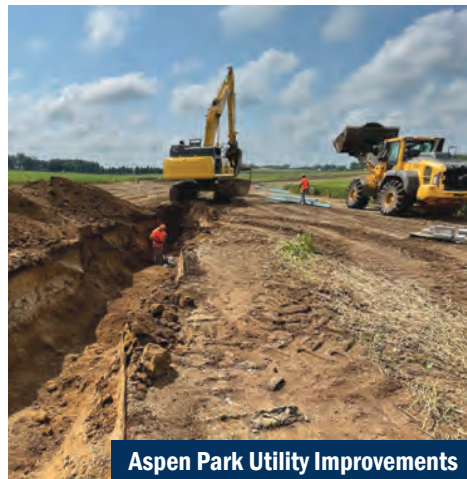
Aspen Blvd. Force Main & Erosion Control
